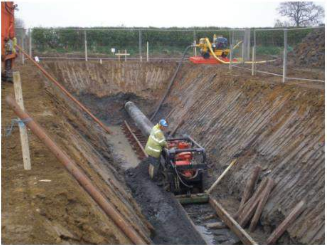
Figure 3-24: Auger Boring at a Road Crossing
