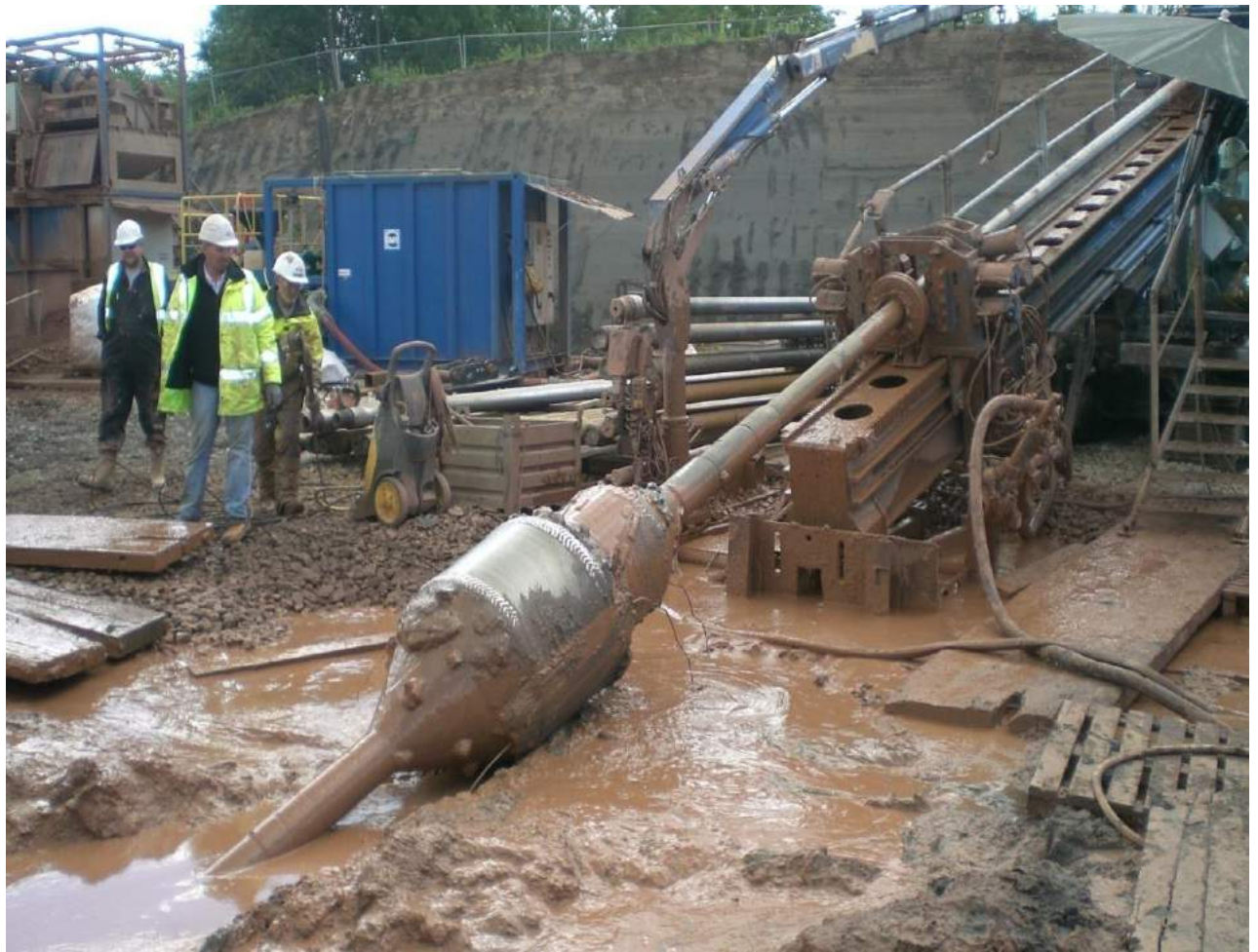
Figure 3-25: HDD Technique
