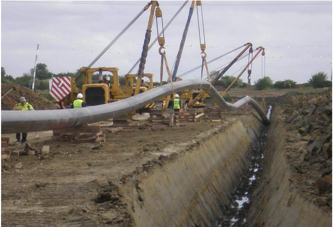
Figure 3-23: Open Cut Technique
