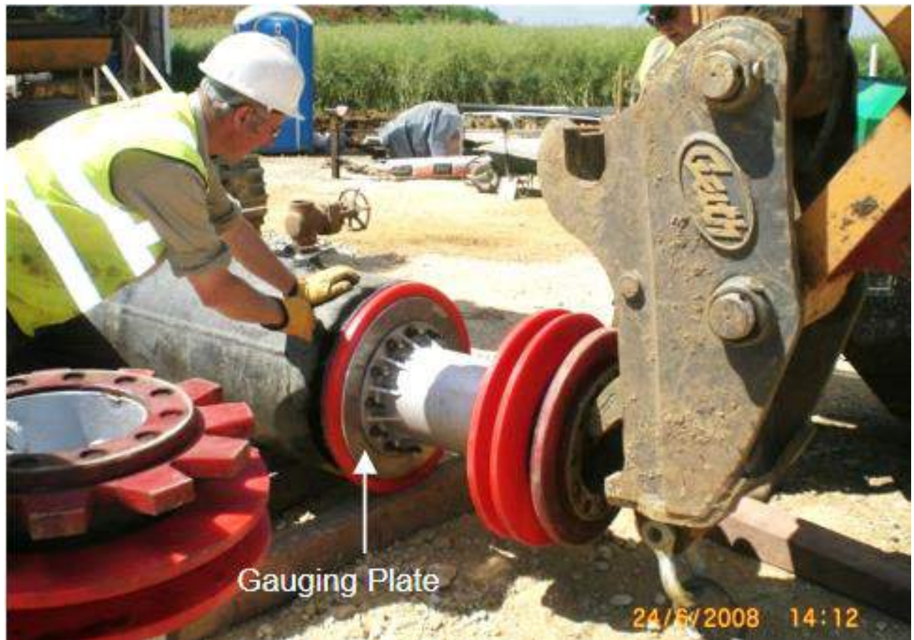
Figure 3-28: Bi-Directional Pig Being Inserted into the Pipeline
