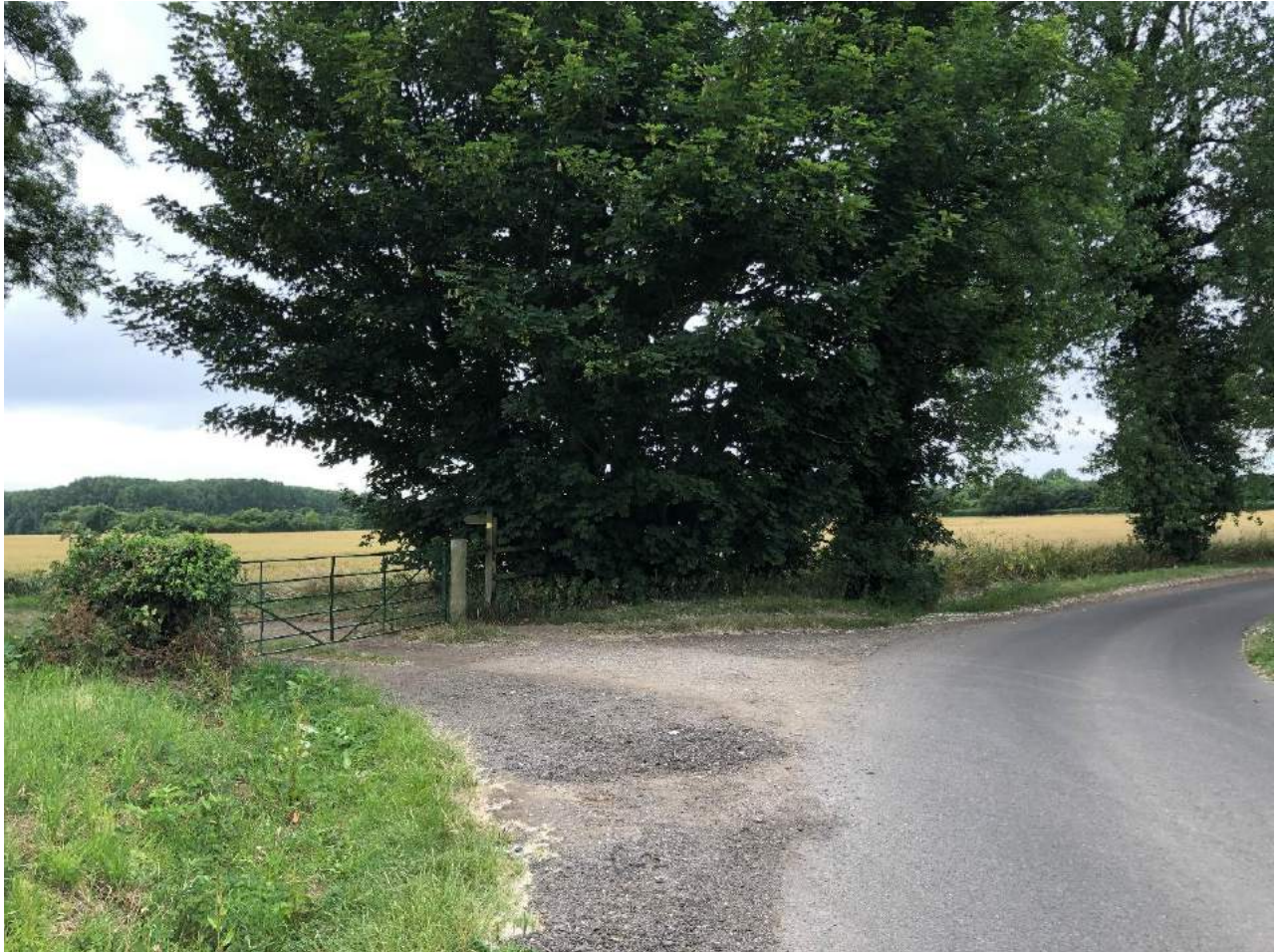
Figure 3-11: Entrance to Block Valve Station No2 (view looking south from public road called Thoroughfare)
