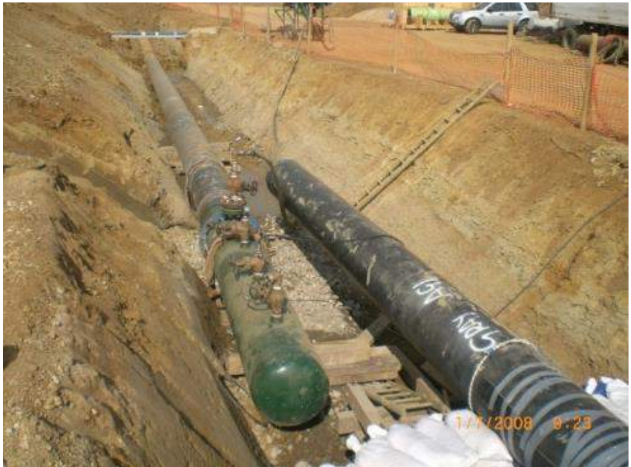
Figure 3-29: Hydrotesting in Operation
