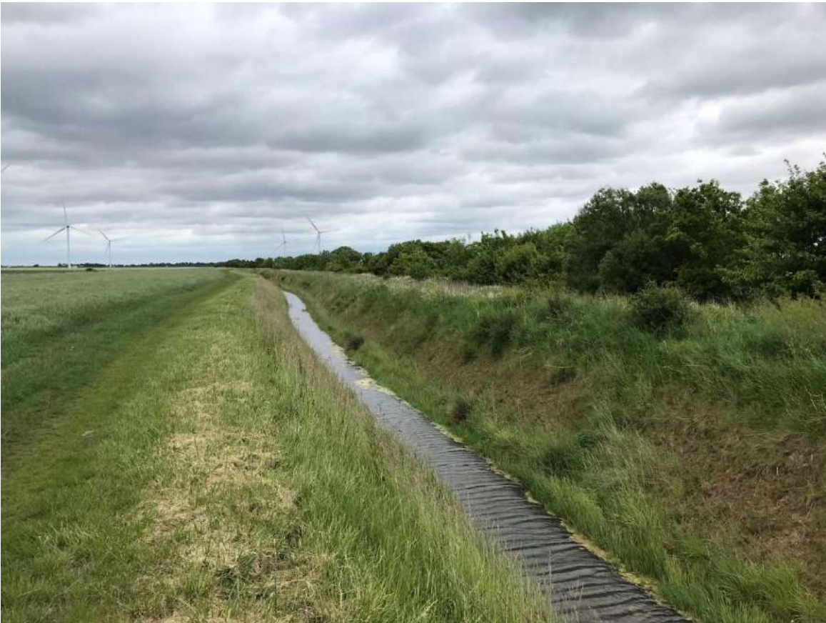
Photograph 11-46: Two Mile Drain (Site 18) View Downstream
