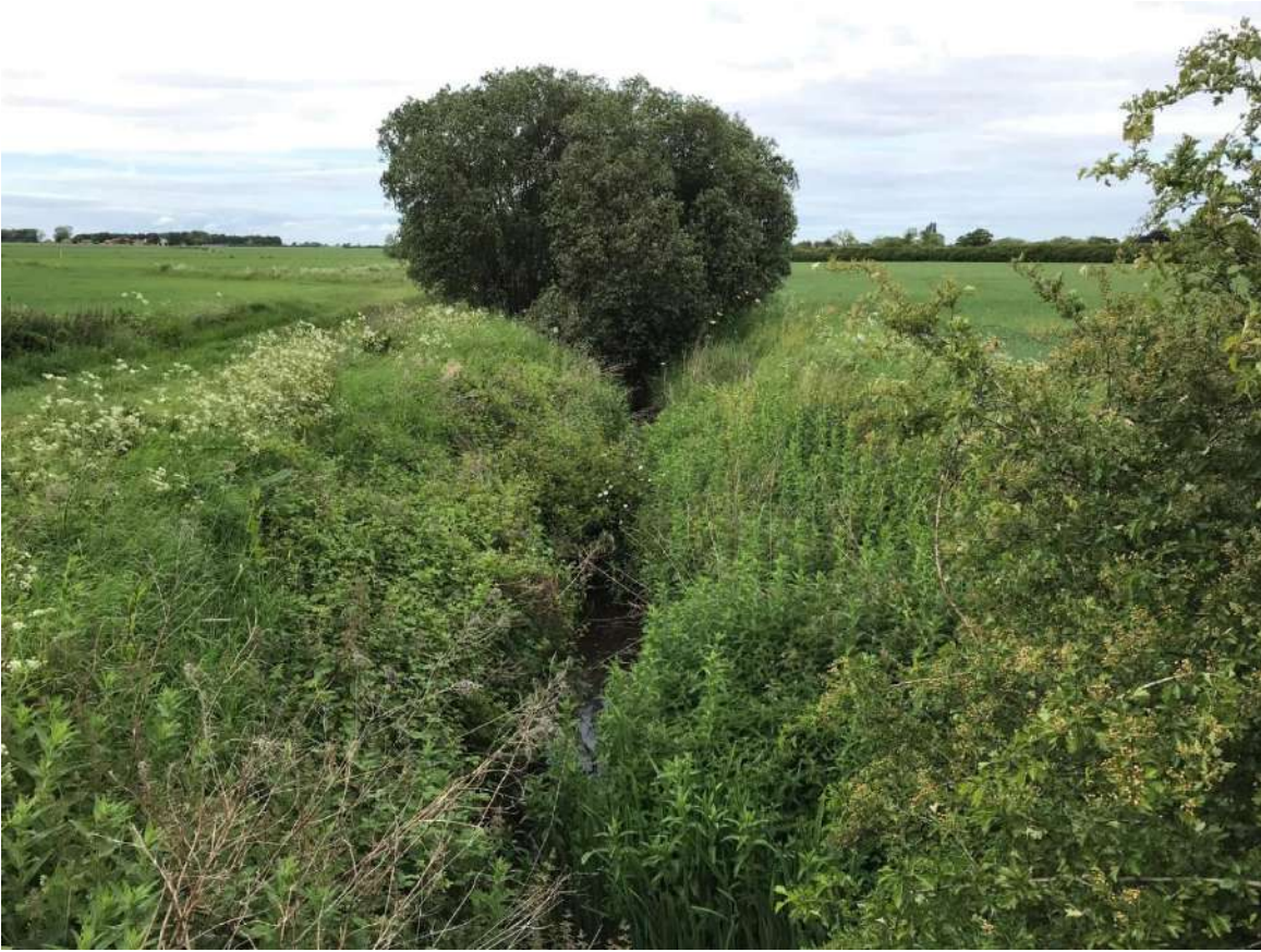
Photograph 11-21: Poulton Drain (Site 7a) View Downstream
