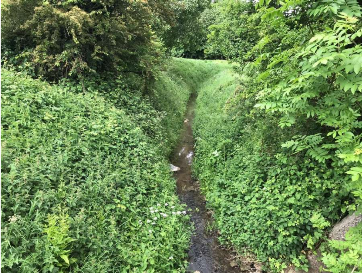
Photograph 11-6: Harborough Marsh Drain tributary (Site 1f) View Downstream
