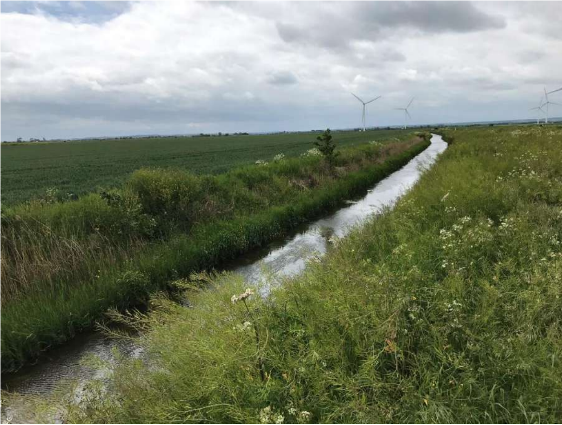
Photograph 11-47: Old Engine Drain (Site 21b) View Upstream
