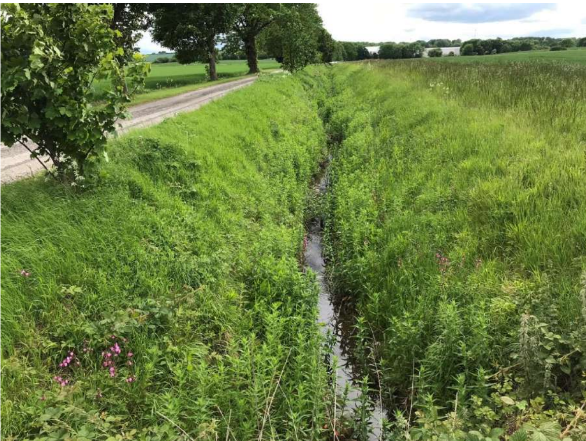
Photograph 11-20: Black Leg Drain (Site 6a) View Upstream
