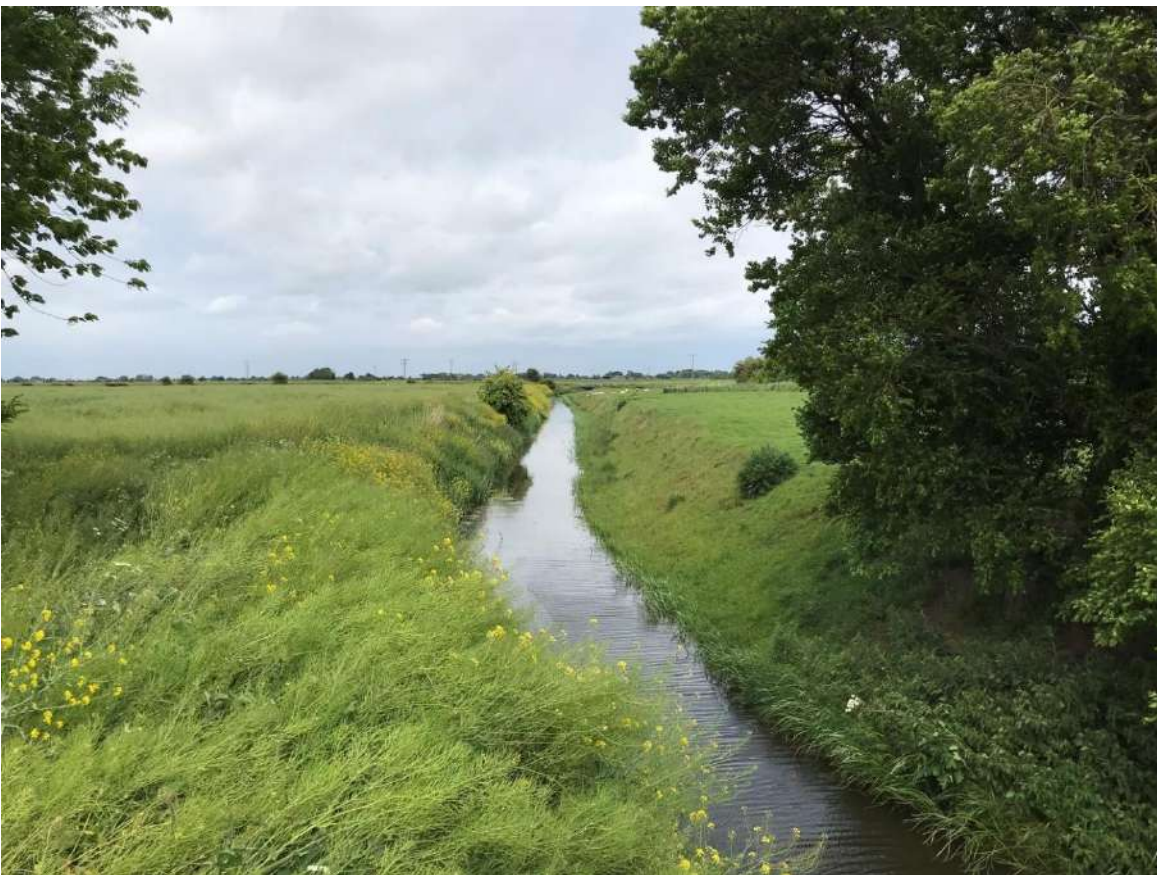
Photograph 11-48: Old Engine Drain (Site 21b) View Downstream
