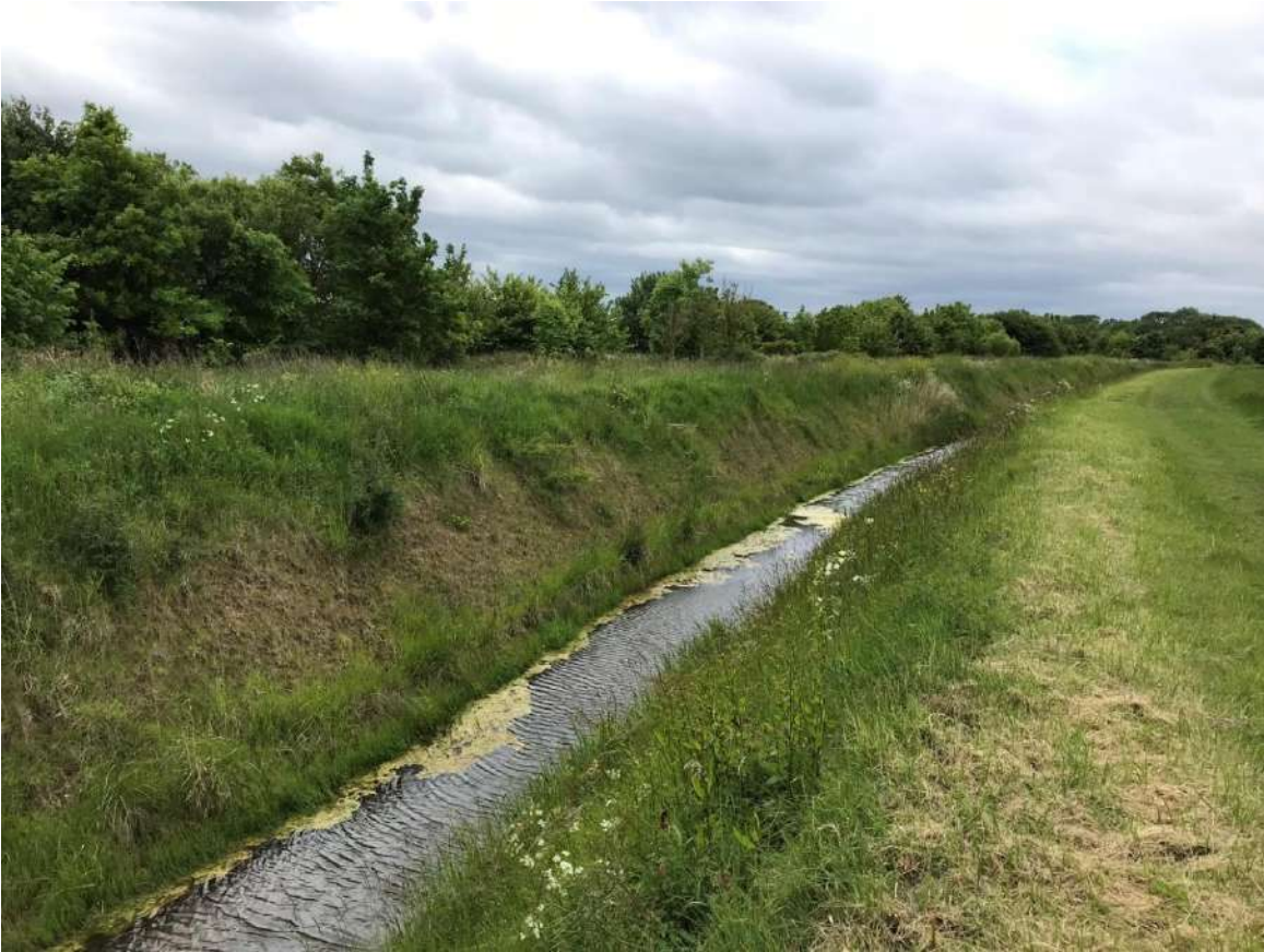
Photograph 11-45: Two Mile Drain (Site 18) View Upstream
