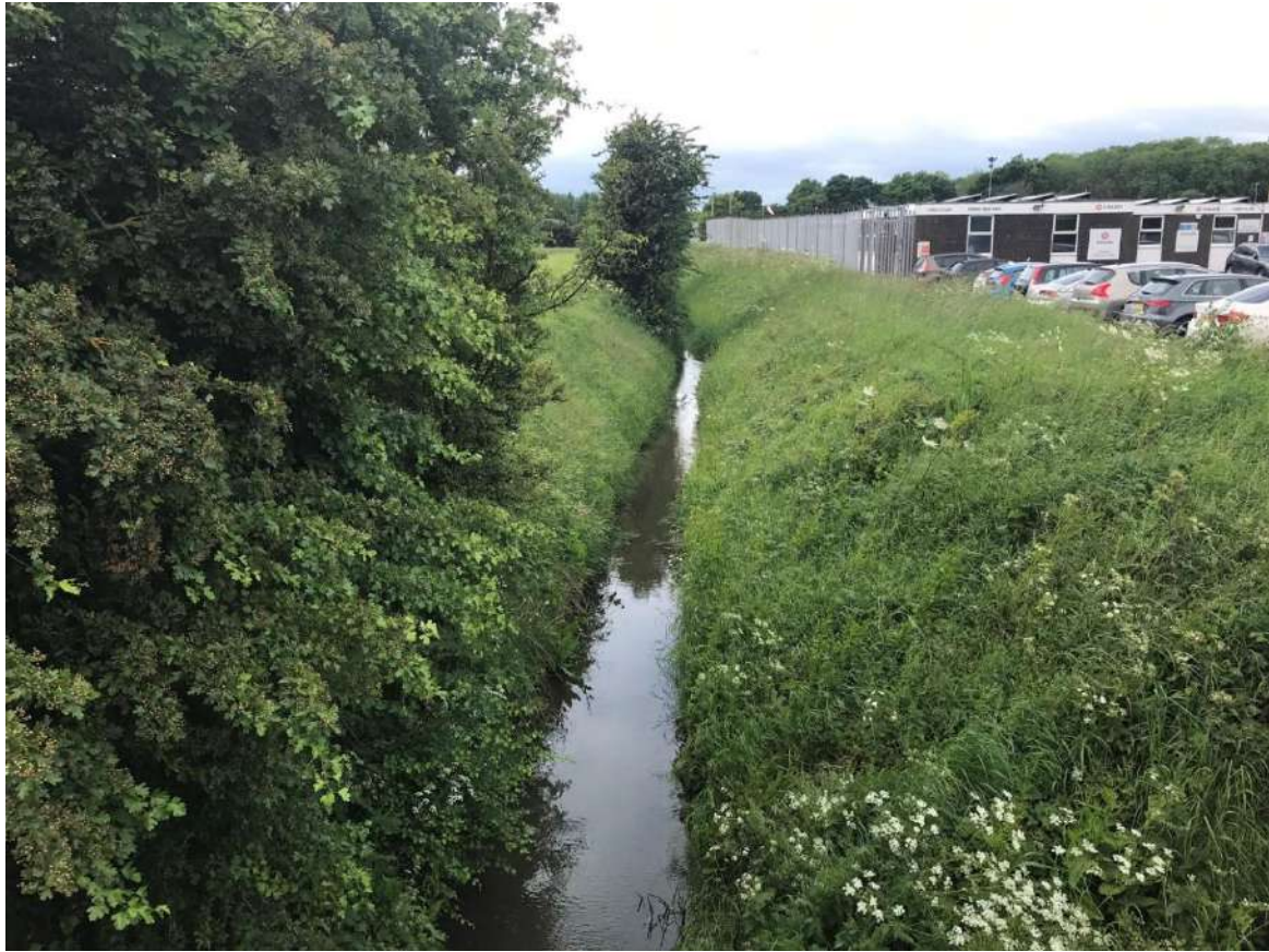
Photograph 11-1: Harborough Marsh Drain (Site 1a) View Upstream
