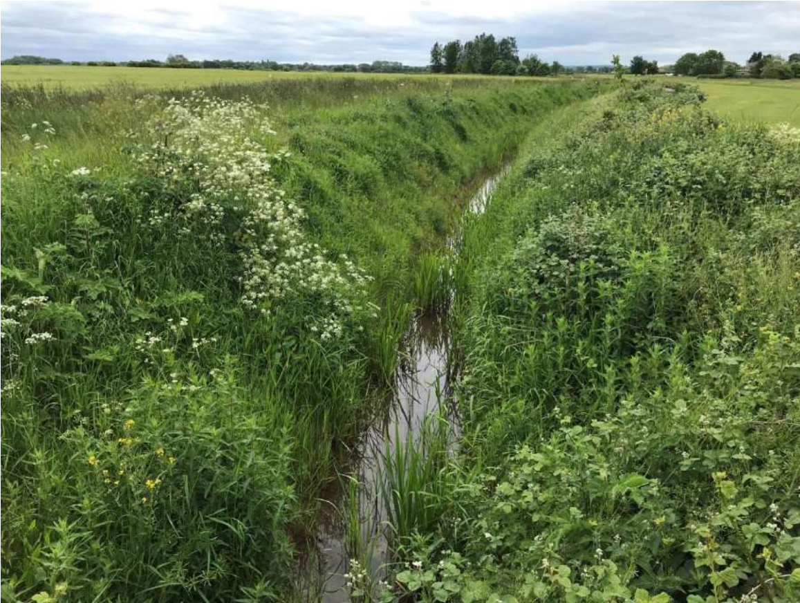
Photograph 11-37: Sykes Drain (Site 14b) View Upstream
