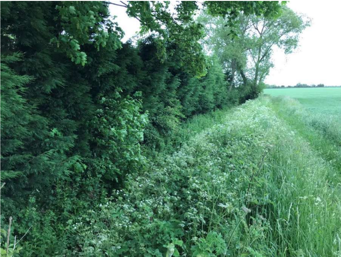
Photograph 11-32: Green Dike (Site 11a) View Downstream
