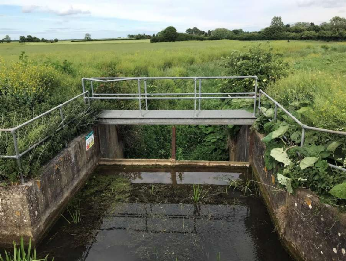
Photograph 11-28: River Ludd (Site 10b) Sluice Structure
