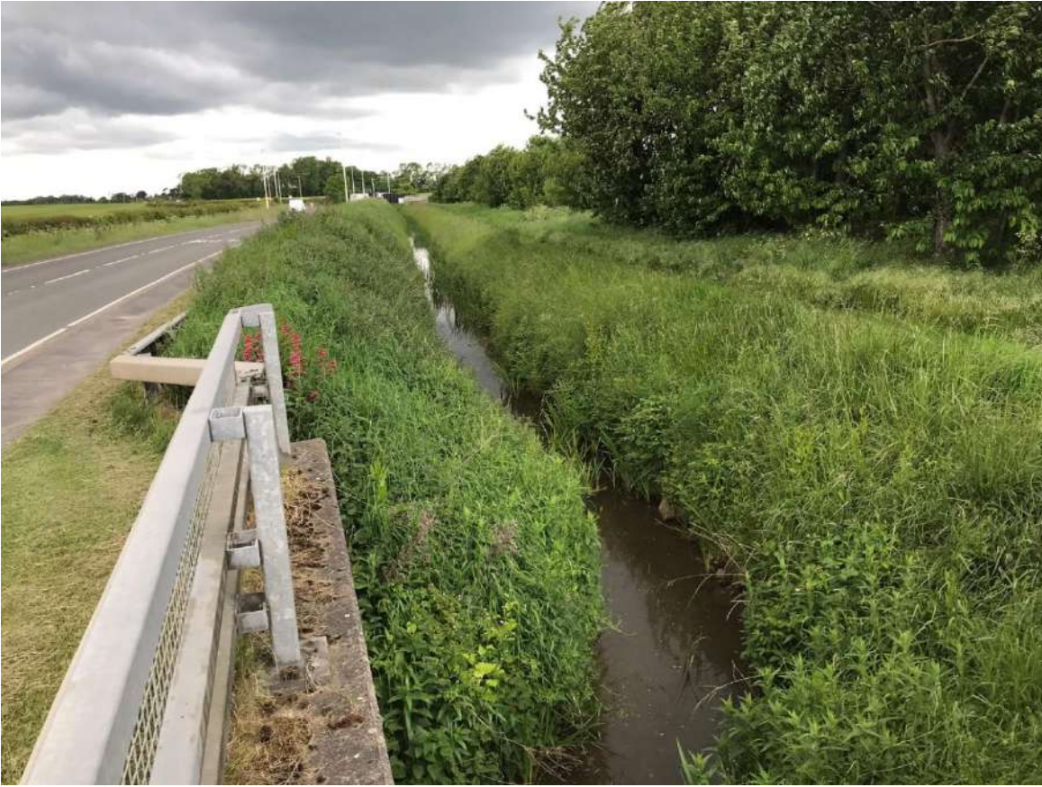
Photograph 11-8: Harborough Marsh Drain (Site 1g) View Downstream
